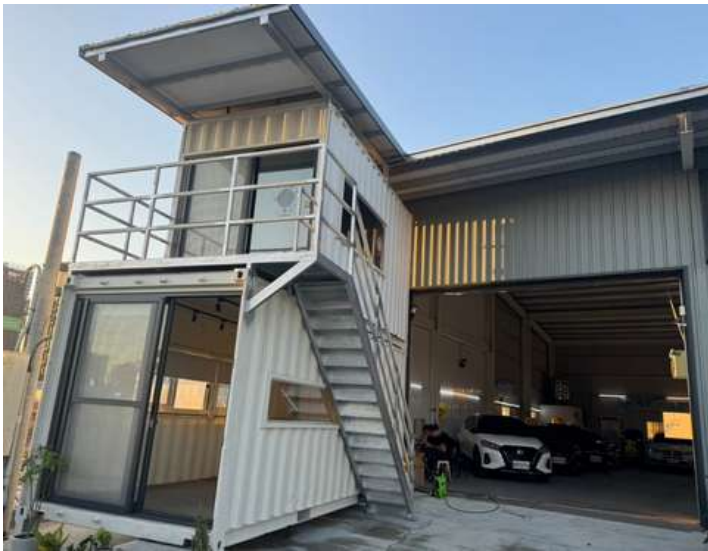
construction site office
